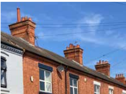
Red brick chimneys
