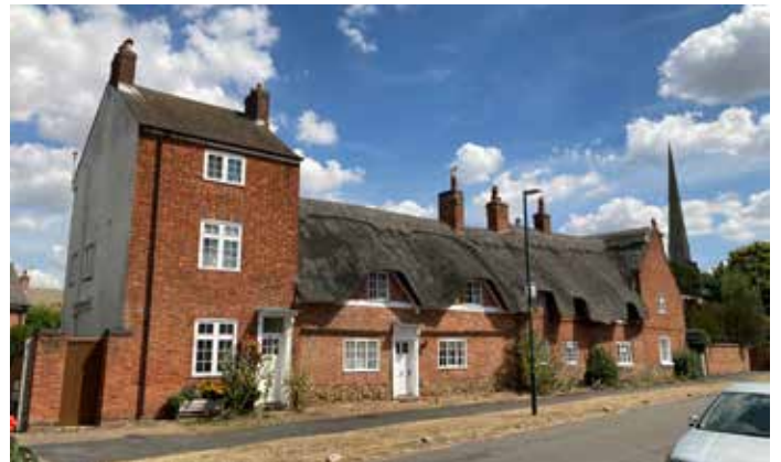
Different buildings unified by brick
