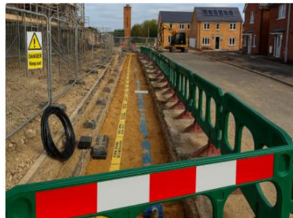
Example of Correctly Installed Service Trench
