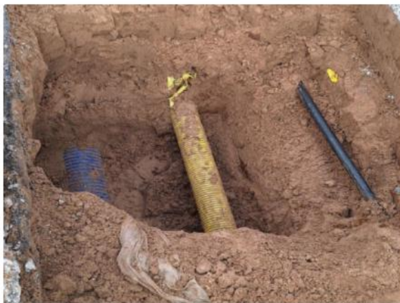
Example of Correct Service Installation.
