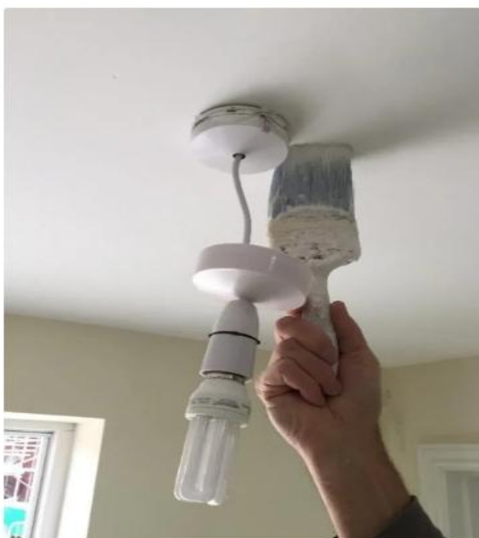
An additional 'paint cover' hides live terminals to allow safe painting whilst light is on
