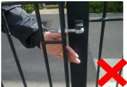
Potential for child to trap and injure fingers between gatepost and pillar
