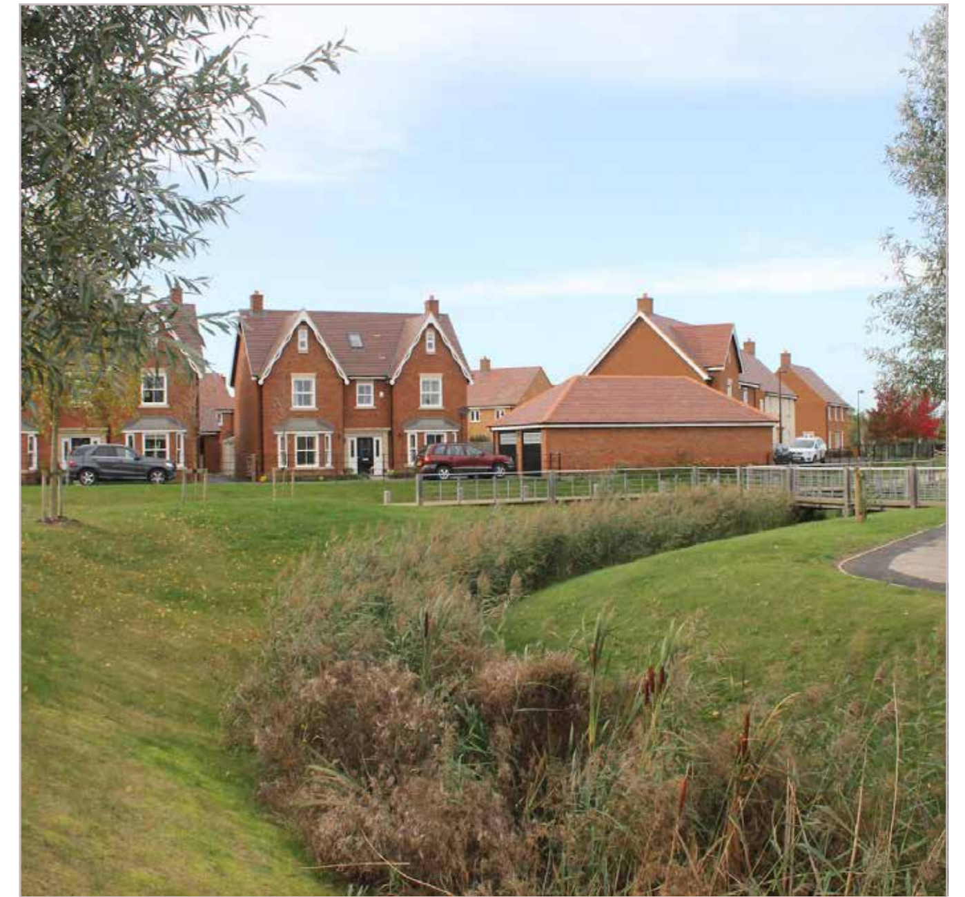
An indicative attenuation basin will help to gradually distribute surface water run off
