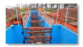
The type of protection used and distance away from the excavation is generally dependent on the depth of the excavation (see section 4.3.2.5), however all excavations, no matter how shallow, that interface with pedestrians or vehicles must have appropriate barriers in place.
