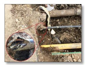
The agreed safe system of work must include the procedures to be adopted if any contact is accidentally made with a live cable, particularly by a machine.
