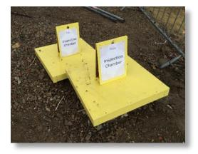
Protected Inspection Chambers with brightly coloured markers to highlight location (e.g. to prevent being damaged by plant, etc.).
