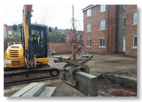
Note: kerb lifting scissor grabs are only suitable for one-off lifting operations. Significant runs of kerbs must utilise a mechanical lifting device which reduces manual handling.
