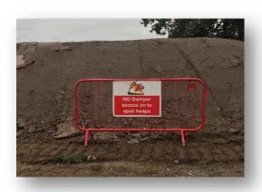
The groundworks contractor, as part of their overall assessment must identify where spoil heaps are necessary to be formed / removed without the use of dumpers e.g., using excavators to drag material up and form the spoil heap.
