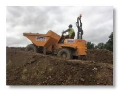
As a minimum, any ramps constructed for dumpers must be set at minimum gradients, well within the safe working capabilities of the dumper, and include bunds at least half the height of the dumper wheel at each side of access routes (prevents the dumper going too near the edge).
