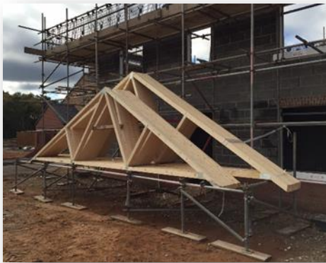
Truss rack attached to scaffold
