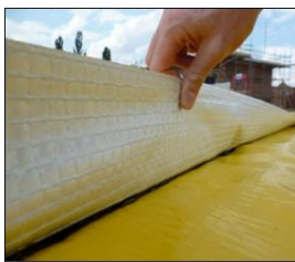
Joints in the membrane are secure
