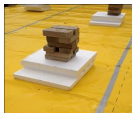
Protecting the membrane after installation
