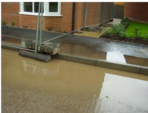
Result of Terram (Drains) not maintained
