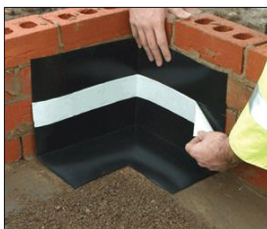
Joints in the membrane are secure
