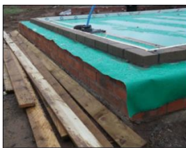
Membrane extending over internal and cavity walls
