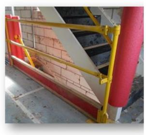
When fitting stairs, there are critical steps in the installation process which must be taken before the stair may be used, even for temporary access.
