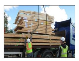
Timber Frame Suppliers must load their delivery vehicles in such a way as to avoid work at height, with either pre-slung loads, accessible from the ground, or draw cords between each panel pack so webbed slings can be attached and pulled through. If such measures are not in place, the delivery must not be accepted.
