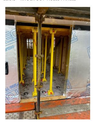
To assist in the installation and dismantling of internal fall protection a 'Knock-out Panel' is left out to provide access from the scaffold and reduce manual handling issues.
