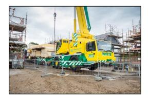
Where materials are craned into position directly from the delivery vehicle, Consideration must be given to the impact on traffic management and access/egress with alternative arrangements put in place before the lifting activity commences.
