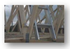
Access for the roof truss installation is normally via the installed perimeter scaffold. Trusses must be temporarily braced (see Section 6.9) as they are lifted into place and again as they are 'spread & spaced' to the required position along the wall plate.
