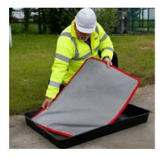
Always use a self-absorbent liner where plastic or metal trip trays are used
