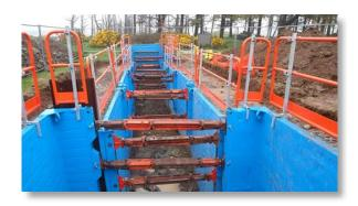
The type of protection used and distance away from the excavation is generally dependent on the depth of the excavation.
