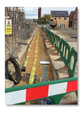
Excavations adjacent to vehicle routes, even shallow ones, must be fenced off to highlight the risk and prevent operatives stepping off or plant driving into them
