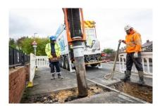
Vacuum excavation can be an effective tool to reduce the likelihood of damaging services or other fragile existing infrastructure, however, as with all works, it requires careful planning
