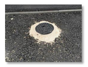
Prior to an area becoming occupied, an inspection of paths, roads, walkways, etc. must be carried out in areas where there is an interface with the customers' homes to ensure that all potential trip hazards have been assessed and appropriate remedials taken, e.g., haunching at manholes, ramps at differing kerb levels, etc.
