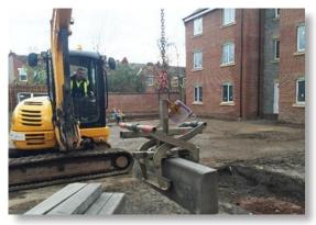
Note: kerb lifting scissor grabs are only suitable for one-off lifting operations. Significant runs of kerbs must utilise a mechanical lifting device which reduces manual handling.
