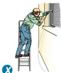
Figure 2a Incorrect - steps side-on to work activity
