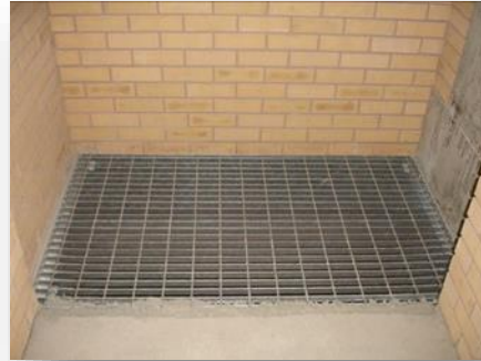
Service risers: fall protection provided e.g., by a secured cover placed over the opening
