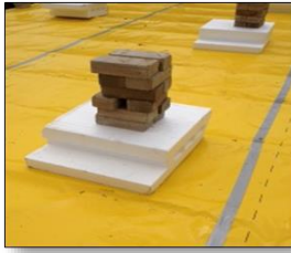
Protecting the membrane after installation
