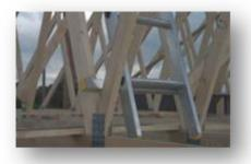
Access for the roof truss installation is normally via the installed perimeter scaffold. Trusses must be temporarily braced (see **section 6.9**) as they are lifted into place and again as they are 'spread & spaced' to the required position along the wall plate.
