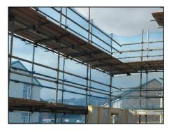
As access is required to the upper lifts of the scaffold before the timber frame erection starts, all Timber Framed scaffolds must have a double internal handrail in place to prevent falls from heights.
