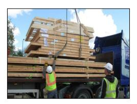
Timber Frame Suppliers must load their delivery vehicles in such a way as to avoid work at height, with either pre-slung loads, accessible from the ground, or draw cords between each panel pack so webbed slings can be attached and pulled through. If such measures are not in place, the delivery must not be accepted.
