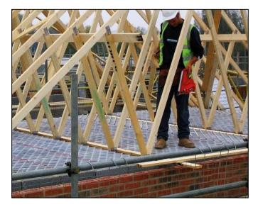
Alternatively, the roof structure can be built a ground-level (space permitting) and then craned into position on the timber frame plot
