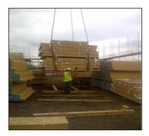
Timber panels and floor cassettes are craned directly into position from the delivery vehicle. However, there may be occasions where this is not possible, and laydown areas are required. This could be on an adjacent plot slab or other suitable area as close to the plot as possible to avoid the need to transport materials on site.
