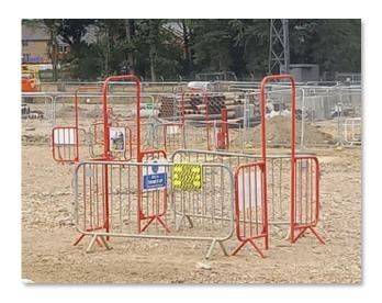
Safe Zones are pedestrian islands comprising of two barriers and two crossing hoops that when positioned around the site allow a haven whilst Groundworks Plant are tracking around.
