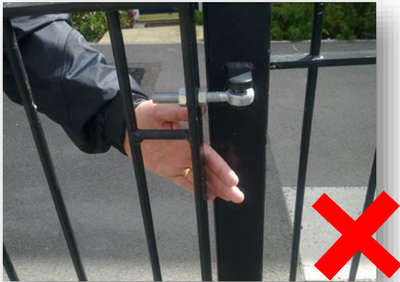
Potential for child to trap and injure fingers between gatepost and pillar
