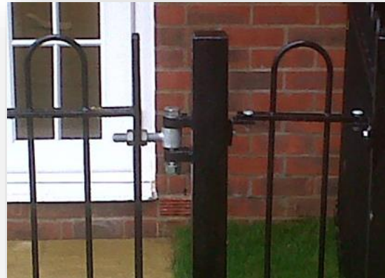
Note the modified hinge with adequate space between gatepost and pillar
