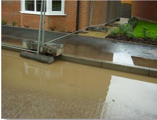
Result of Terram (Drains) not maintained
