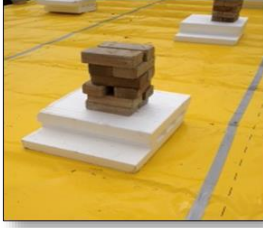
Protecting the membrane after installation
