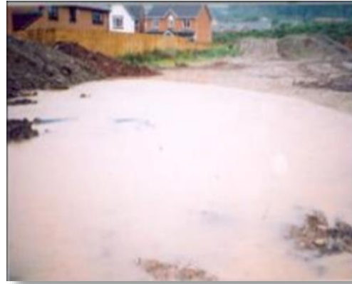
Excessive/unnecessary soil strip
