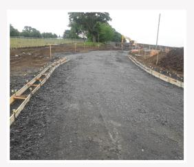
1 The SiteM must ensure capping and sub base material is installed as per specification. The roads inspector must be notified at the correct time and encouraged to regularly inspect the road construction process. The SiteM must ensure the roads inspector approves the formation once dug and exposed.
