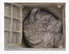
Placement of gully guards (or standard protection, e.g. straw and terram) in all gullies during construction and inspected, replaced / cleaned regularly.
