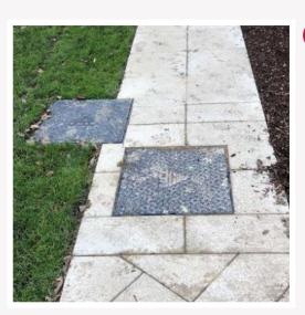
2 Layouts for manhole placement should be followed however, consideration should be given to locating manholes not within vehicle track lines on driveways, outside of front doors and located fully in the garden or footpaths. Local adjustments can be made to accommodate the considerations highlighted above.
