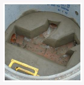
1 Groundworkers should bench their manholes as construction proceeds and certainly prior to the sewer becoming live, this will help prevent blockages due to snagging of waste on rough benching.
