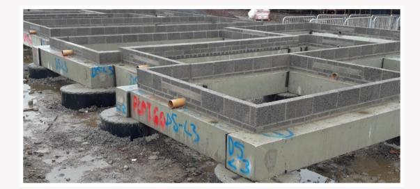
1 This type of foundation is similar to a piled foundation but the head supports a preformed beam.
