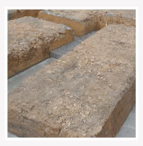
4 The SiteM must ensure levels are checked at key stages of direction in the build. Ensuring checks are undertaken prior to substructure brickwork and the level of foundation brickwork prior to floor. Concrete overpour must be avoided in any pour.
