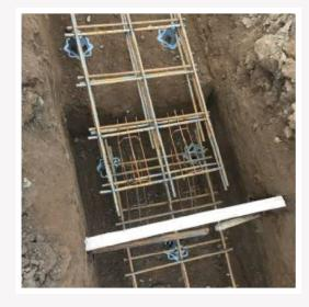
3 Steel reinforcement is generally required as per design and should specify the steel type, gauge and orientation. Proprietary supports for reinforced steel should be used for a 75mm minimum cover and should be supported every 1m maximum staggered centres and spacers should be staggered to avoid planes of weakness.
