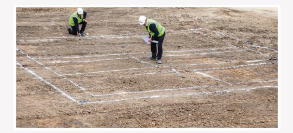
Marking out of foundation locations should be undertaken by a Setting Out Engineer using a consistent source for coordinates. The coordinates will be provided by TW Technical. SMT should check the handing and house type prior to excavation.
