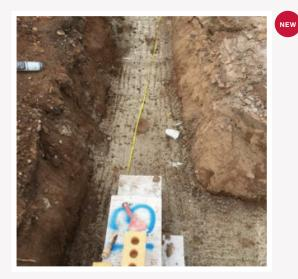
**2** The wall should be positioned on the centre of the foundation.
