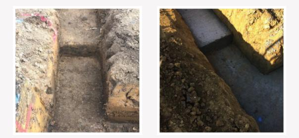
**2** The finished height of concrete after pour must be level.
