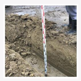
1 The appointed Structural Engineer should attend and agree bearing levels with the Groundworks Supervisor and SiteM. Foundation depths should be checked against engineering drawings and the foundation zoning plan. This is also a key inspection stage for a warranty provider.
