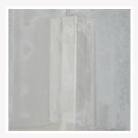
**1** Gyproc corner tape should be used for external angles and splayed internal angles.
