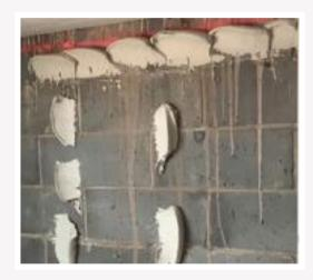
2 Dabs should be applied in a regular pattern in accordance with BS 8212 and BS 8000. Part 8 to give a minimum area of contact between board and background of 20%.
