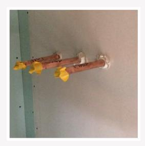
**1** All service penetrations through the plasterboard should have a perimeter seal to prevent air leakage and prevent ingress of fire into the cavity.
