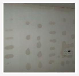
4 Mould growth and moisture migrating through to the plasterboard surface can occur when plasterboard is applied onto wet masonry backgrounds. This can be evident during the construction process however, mould growth can also occur once a property has been occupied by a homeowner.
