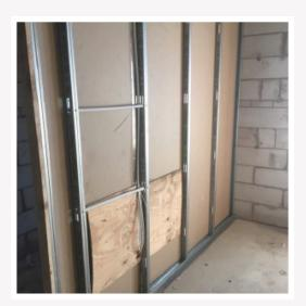
4 Either metal or timber studs may be used dependant on plot design. Sheeters must follow the British Gypsum guidance on fitting plasterboard to either system.
