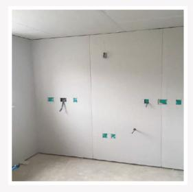
Plasterboard should be free of damage. Plasterboards should be delivered, fitted as soon as possible to ensure they are not stored outside and exposed to the elements.
