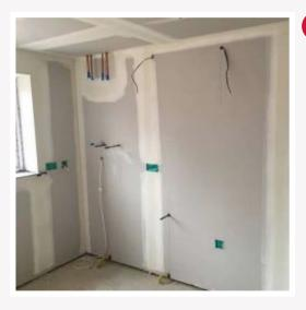
2 Joints must be sanded using a sander from floor to ceiling and the finish must provide a smooth level surface for paintwork to be applied. Ensure a mask is worn and an extractor used to reduce the level of dust as per HSE Manual Guidance.
