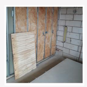
**8** Acoustic insulation is usually installed by the Drylining Contractor and should follow the plot specific design in line with the product specification.
