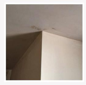
1 Before skimming, all surfaces must be dry, clean and free from loose material. Plaster should be recently and thoroughly mixed using clean water, opposing walls should be skimmed first to achieve the best finish for internal corners.
