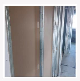
**3** Plasterboard must be fixed securely to the metal stud and floor track.
