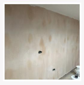
3 Plasters must only be applied where backgrounds are not frozen or will remain at 2 degrees or above until dry. Ambient and background temperatures must be maintained above 5 degrees until fully dry to apply ThistlePro DuraFinish.
