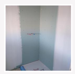
Where shower trays meet masonry walls the plasterboard should be as snug as possible allowing wall tiles to be fitted. For tiled areas, studwork must be at max 400mm timberstuds and 300mm for metal studs.
