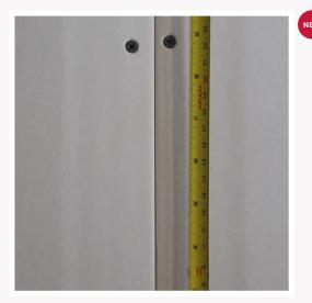
4 Plasterboard layers should be screwed at 300mm centres except at external corners where spacing centres decrease to 200mm centres.
