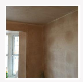
Plaster should cover walls from ceiling to floor to give a smooth, consistent finish. In shower rooms, it must cover the plasterboard down to where it meets the tray and be a minimum of 2mm thick. Plaster should be applied in two applications wet on wet. Plaster should be given a minimum of 24 hours to dry before mist coat begins.
