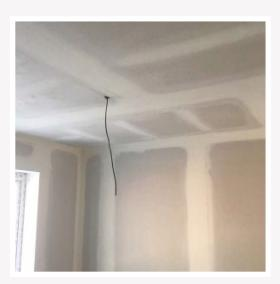
3 Three applications of jointing compound should be applied. The compound must be dry before the next application, feathering each out beyond the previous application. Sand each joint as required to remove any imperfections.
