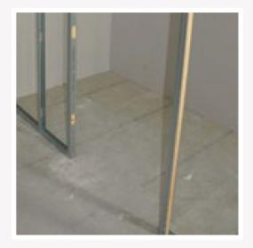
**5** In line with BS 5234 for Light Duty door openings best practice is to reinforce metal studs with timber.
