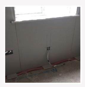
2 Plaster board should have a solid dab along the bottom of sheets.
