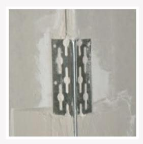
**1** The correct external beads must be used in line with TW specification.
