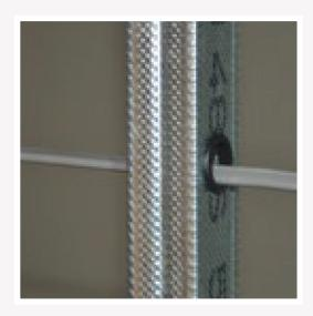
1 It is very important that any holes, through which services pass, in metal studwork are protected by rubber grommets to prevent the pairing away of insulation on electric cables.
