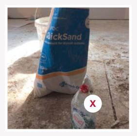
4 It is important **not** to use any additives which will compromise the performance of Gyproc jointing products in terms of reduced strength and sanding characteristics. Clean water only should be used for mixing joint materials. Ensure bags are fresh, unopened and not damaged.
