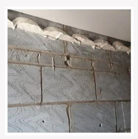
3 Minimum clearance of 100mm at ceiling / floor junction to prevent micro cracking 25mm elsewhere.
