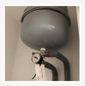
**2** Pipework for cylinders to be installed neatly. Pressure gauge on cylinders must have easy access for viewing.
