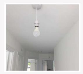
2 In the event, a pendant light clashes with an opening door the flex should be reduced or a batten holder used.
