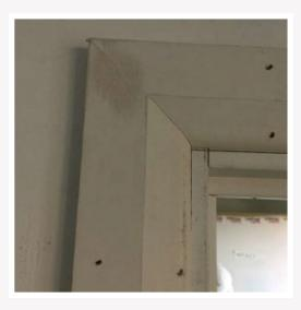
**3** All facings should be neatly cut and mitred with joints glued and sanded. Ensure that an even perimeter is allowed between the edge of the door lining and the architrave allowing room for the door hinge to freely work and adjustment with cranking tool.
