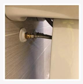
Pipes to be placed to be aesthetically pleasing and hidden by the pedestal as much as possible. Pipe collars should be fitted to soil and water pipes where required to provide a tidy finish.
