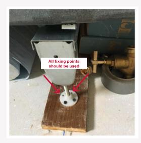
The bath legs should be secured to the floor using the fixings supplied with a timber support to stabilise (minimum 90mm x 22mm softwood). It is best practice once water is on to fill the bath and assess any adjustments that may be required due to movement.
