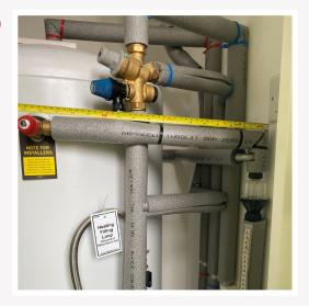
1 All pipes within 1m of the tank, or to concealment should be lagged.
