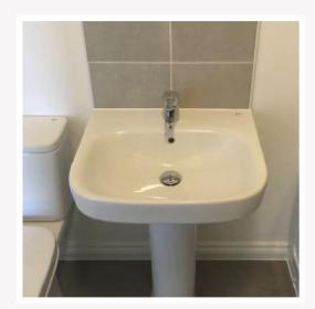
2 Basins must be fitted with the appropriate pedestal in correct alignment between the bowl and the waste outlet. The perimeter of the basin should be fully sealed with no gaps using the TW recommended sealant.
