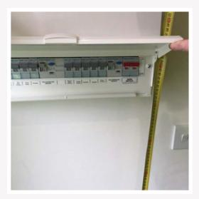
3 Consumer unit circuits should be labelled so each isolator can be identified and include commissioning label (dated and signed).
