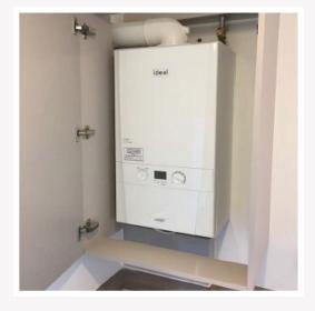
3 Boilers and radiators should be filled with cleansers, inhibitors added and tested at this stage and all pipework checked for leaks.
