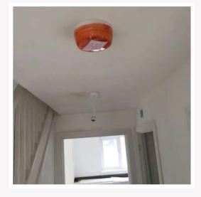
3 Smoke detector should be installed as per drawings and the dust cover should be left in place until the customer moves in. Customer should be advised that the detector should be protected where there is ongoing work which could generate dust.
