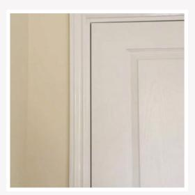
2 Equal 3mm margins should be maintained to all sides of the door to allow air flow. There should be a 10mm undercut to the finished floor level and 22mm undercut to unfinished floor level in line with building regulations.
