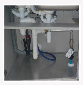
1 Under sink pipework should be neat and clearly labelled for customer information.
