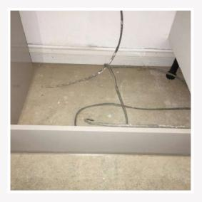
2 Skirtings should also be fitted behind kitchen units to minimise sound passage and air leakage.
