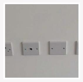
All outlet boxes must be cleared of plaster and debris and when more than one are fitted together at a distance of 75mm (one box width) between and each box must be fitted plumb.
