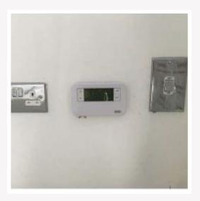
2 Thermostats should be fitted as per the heating design to provide zone controlled heating.
