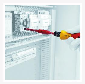
1 Consumer unit manufacturers state torque settings for their terminals including main switches, Miniature Circuit Breakers (MCB) and Residual Current Circuit Breakers (RCCB). Installing contractors must ensure they are being installed in accordance with these requirements by using a torque screwdriver. Ensure there are no gaps between MCBs and Residual Current Devices (RCD). All consumer units must have their connections checked at the time of installation.
