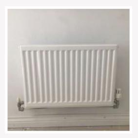
2 All radiators must be level and securely fixed with pipework concealed behind the radiator. Radiators should be secured in line with HSE Manual Guidance.
