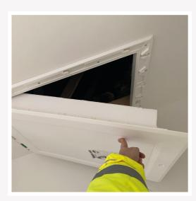
**2** Loft hatch to be installed as soon as practically possible to prevent moisture build up in loft space.
