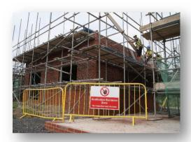
The approach to setting up a 'Scaffold Exclusion Zone' will differ depending on the plot e.g. route of traffic management, telehandler off-loading area, etc. However, a simple assessment during 'pre-call-off' or 'prework' checks by the Site Management Team and Scaffold Supervisor can identify the most prominent location for the warning signs, to achieve maximum exposure.
