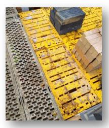
**Note:** All scaffolds must be erected to minimise the internal fall distance, including the installation of proprietary decking systems (i.e., TRAD, RHINO or M&G decking systems)
