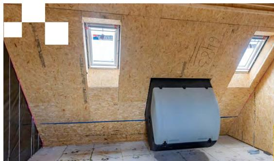
We are testing a roof-mounted air-source heat pump (ASHP) at our site in Sudbury. This can help to mitigate issues with constrained external space. The ASHP is supplied within a sealed Hydrotop unit, to limit noise and air leakage. The unit includes an access hatch allowing commissioning and maintenance to be completed from inside the plot, avoiding working at height.
