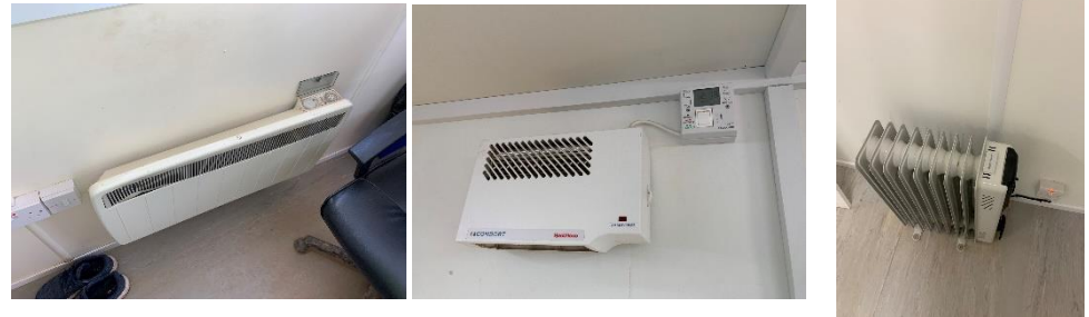
Above: Various electric convection, fan, and oil filled radiators used in the cabins. Below: Basic thermostats and analogue timers were rarely used to optimal effect.
