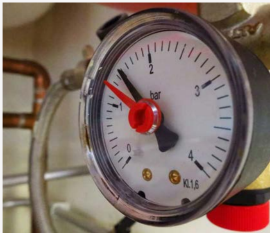
PRESSURE GAUGE SET TO 1.5 BAR
