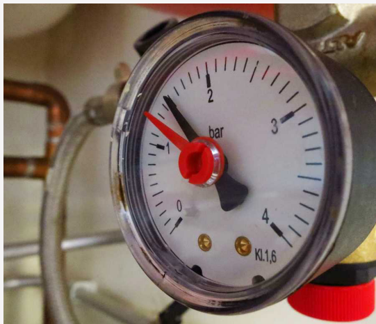
PRESSURE GAUGE SET TO 1.5 BAR
