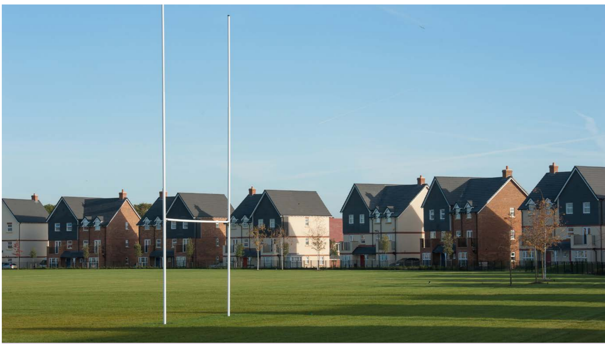
Our Great Western Park development in Didcot
